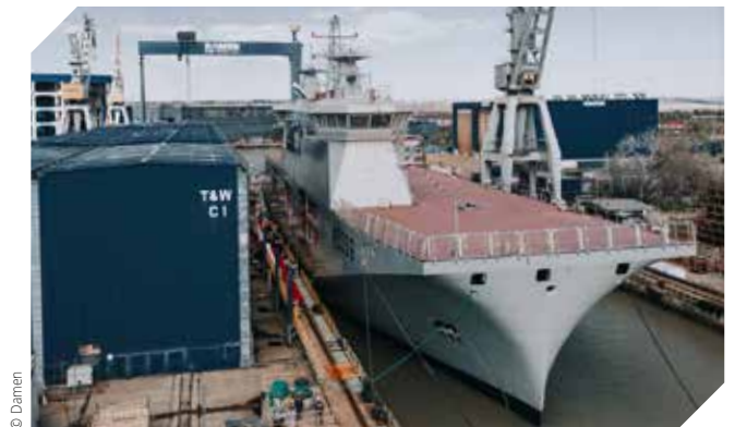
The future Portuguese amphibious drone carrier under construction at Damen in Romania.
